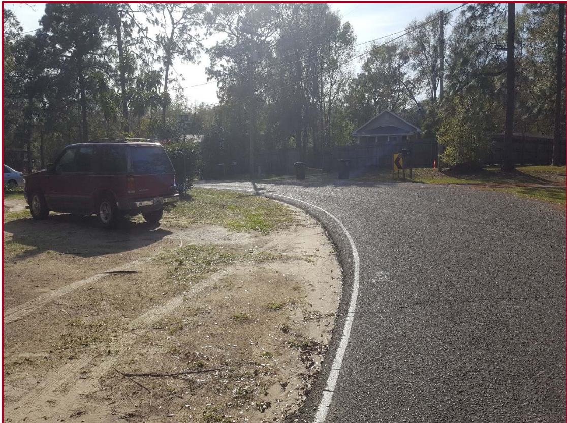
FIGURE 3D: EXISTING SITE CONDITIONS ALONG MARGO STREET NEAR SOIL BORING SS-9 (FACING WEST)
